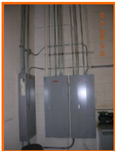
240/415 Volt Panels along with 110/220 Volt Panels
