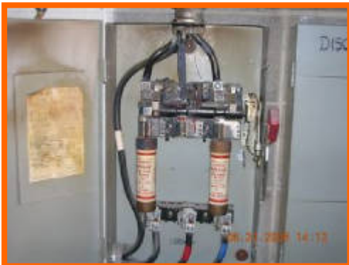
Service panel disconnect with "B" phase wire burnt off.
