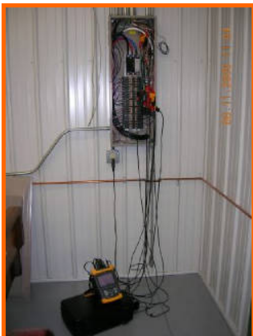
Capture and record events at the main panel feeds or an individual circuit.
